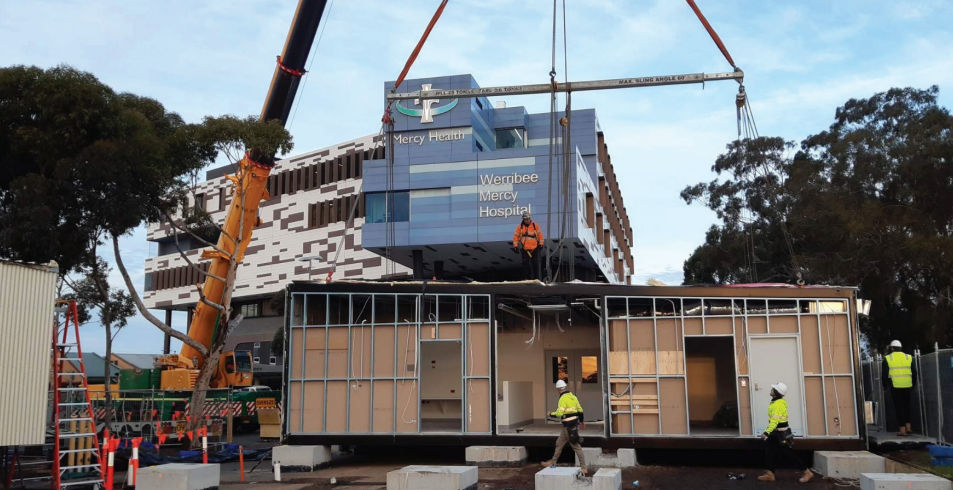
The new Short Stay Unit, enabling more Emergency Department care, is craned into position at Werribee Mercy Hospital.
